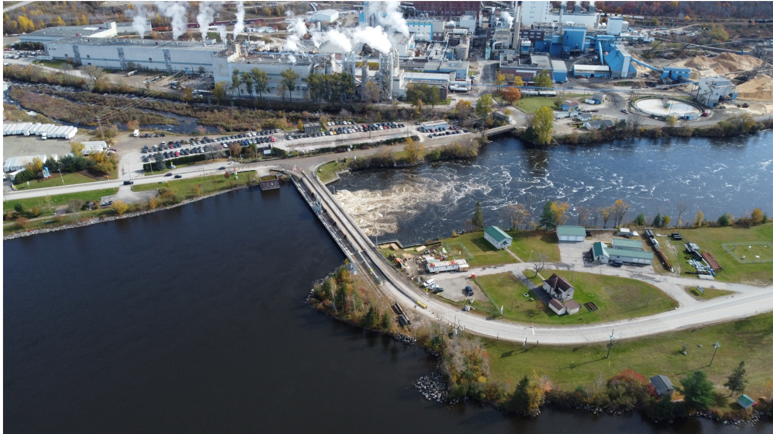
Timiskaming Quebec Dam – October 2020
